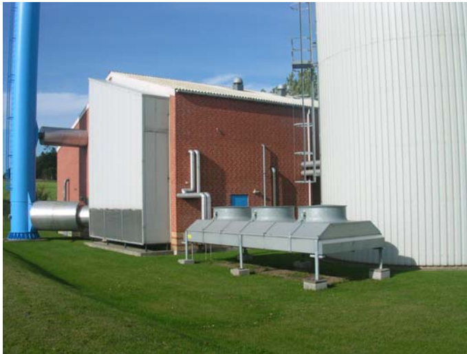
Figure 4: Some of the CHP-plants have cooling towers, making these plants more available in the balancing markets.
