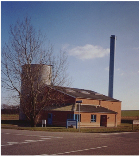
Figure 2: Danish CHP-plants are made flexible through big thermal stores and high CHP-capacity. Typically with a heat capacity of the CHP-units around the average demand of heat in winter. In this picture is shown a 2 MW-el CHP-plant.
