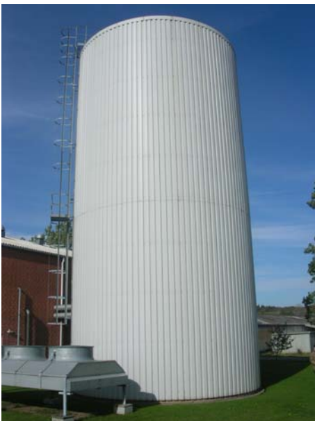
Figure 3: The big thermal stores at the Danish CHP-plants are equal to around 200 m 3 per MW-heat on the CHP-units.
